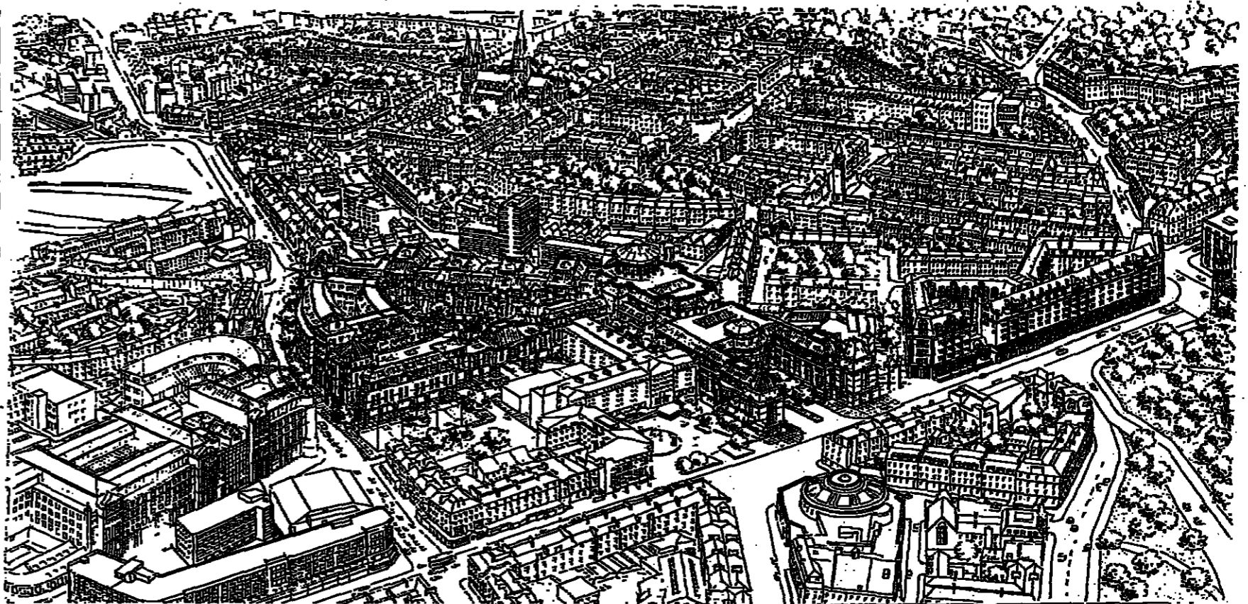
An impression of the proposed Lothian Road development in Edinburgh which includes a conference centre (see Page 2)
